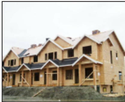
A new townhome complex currently being built using chipboard.
