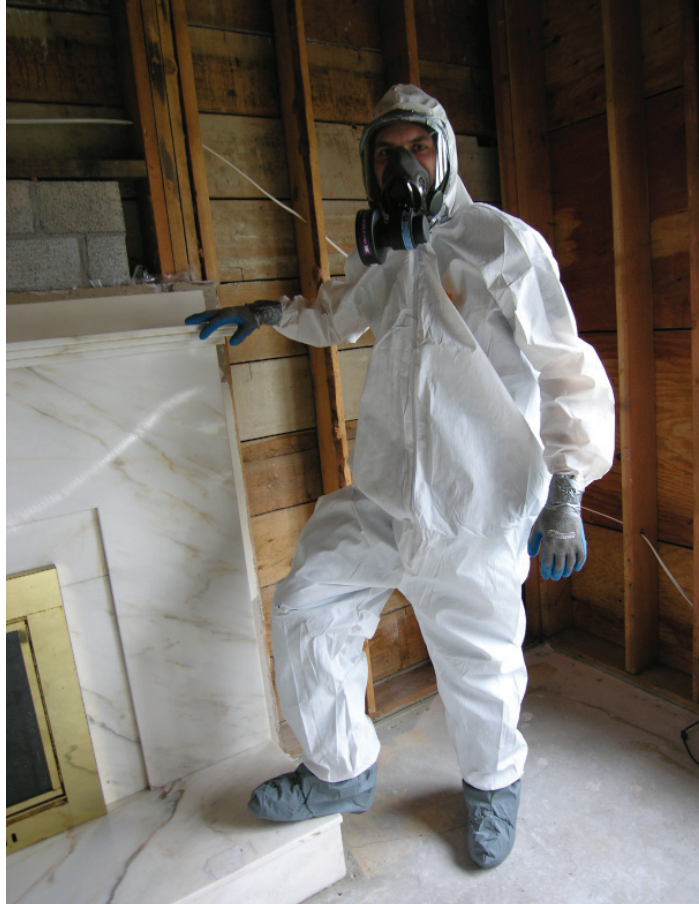
Figure 7. Suggested protective ensemble for restoration worker at a post fire scene. The combination of the disposable suit + PAPR (HEPA + acid gas/organic vapor cartridges) + gloves + safety footwear taped together forms a sealed unit. This ensemble is common to other remediation work including asbestos removal and bloodborne pathogens and must be selected and assembled with consideration given to ease of removal to prevent spread of contamination to underclothing and the skin.
