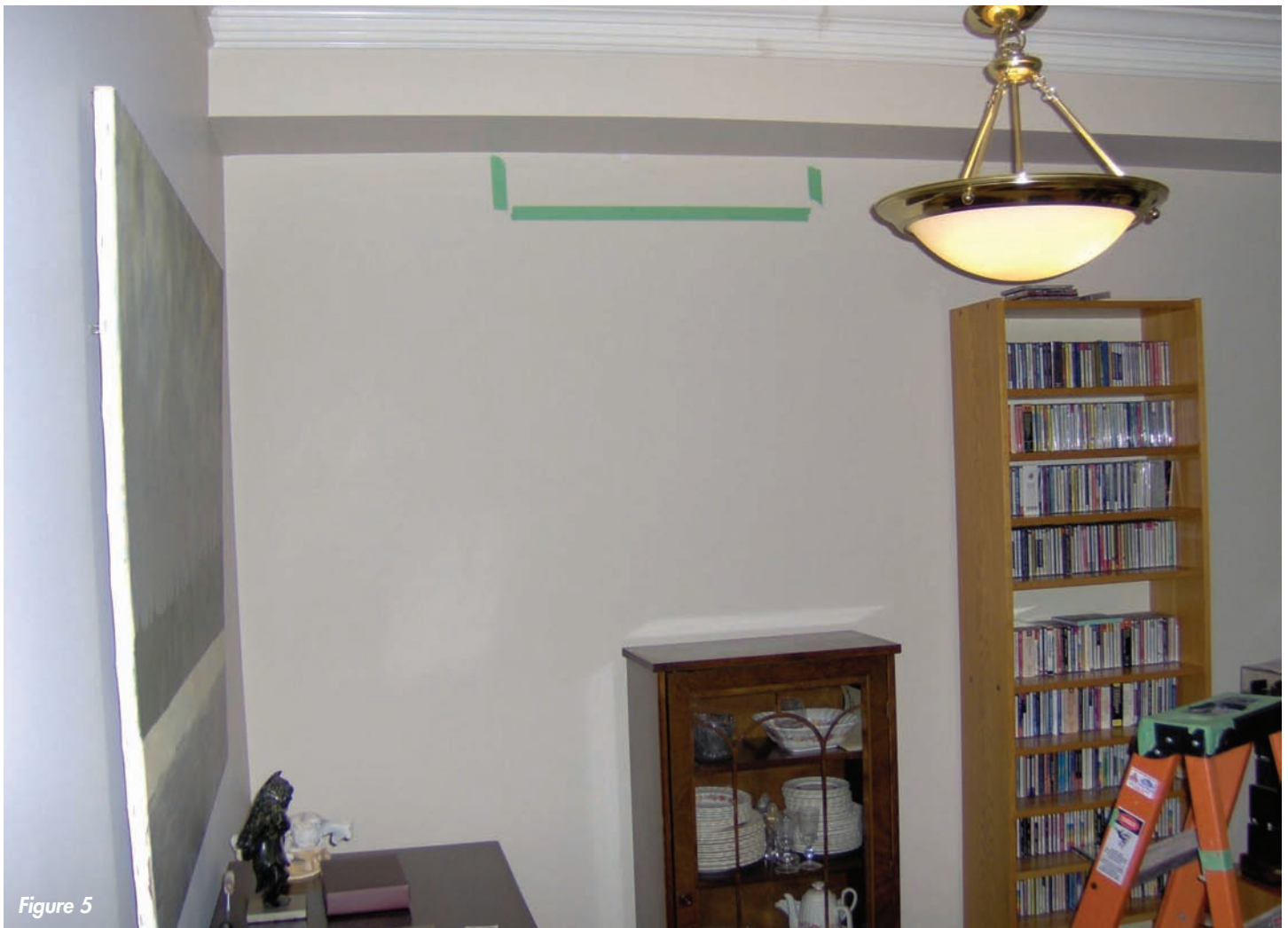
Figure 5. Wall showing extent of migration of water from the ceiling. Surface sampling indicated mold contamination in the area wetted located above the tape and lack of contamination in areas of the wall located below the tape that had not experienced wetting.
