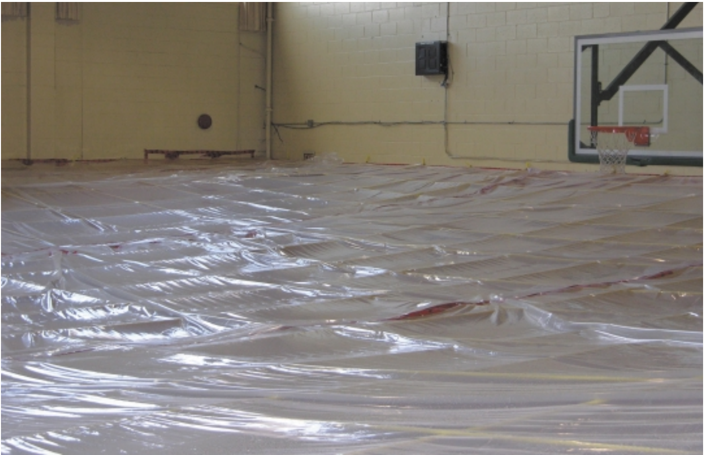
Figure 4. The network of ropes that held up the sheet poly to create the ceiling of the containment.
